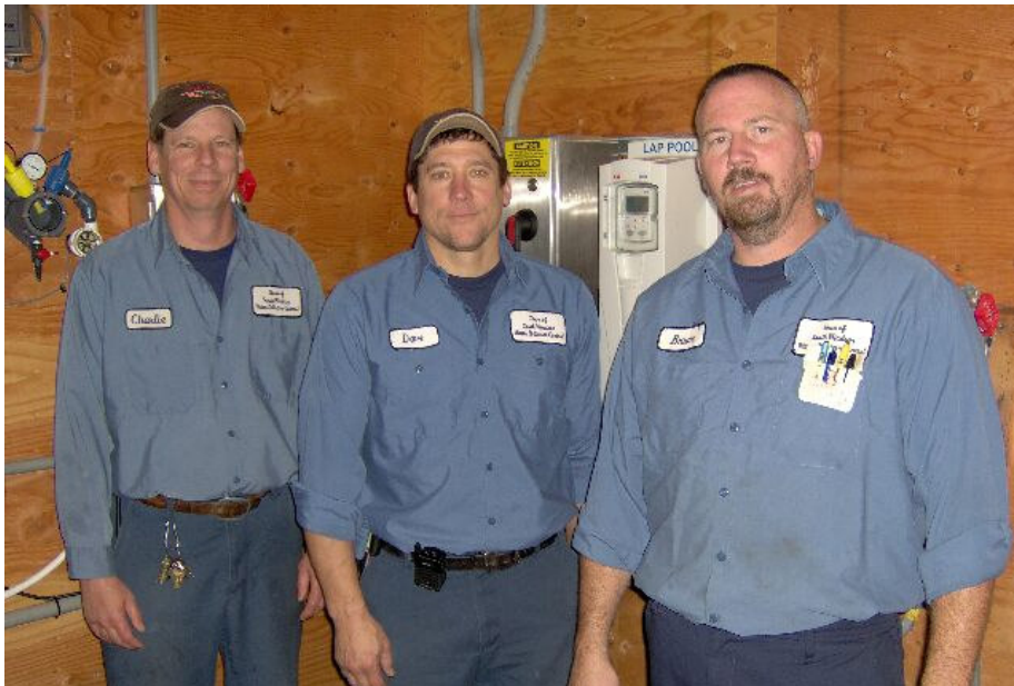
Charlie Albert, Dave Geng, and Bruce Lundie (left to right) handled the installation of all the ABB drives, operating the filtration pumps for the three pools in Windsor, CT.
