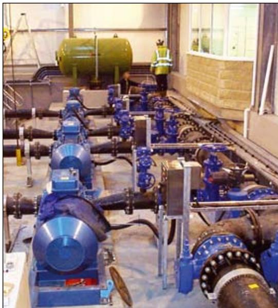
The treatment works' four drives pump 5 million litres and 10 million litres per day in adjustable combinations
