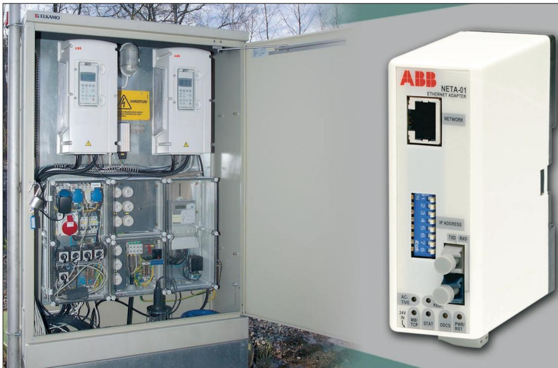
Increasing wastewater treatment requirements prompted Larsmo municipality in Finland to take action to combat the problem of stormwater leakage into its sewer system. A remote monitoring system was installed at a pumping station to allow operators to monitor the volume of fluids being pumped and therefore detect when stormwater leaks into the system.
