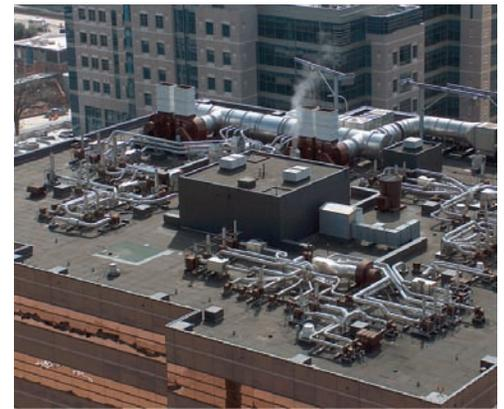
**Feigin’s existing roof was riddled with small fans from original lab exhaust. The project team was faced with the relocation of existing exhausts, affecting a total of 125 hoods within the building. Photo: FKP Architects**
