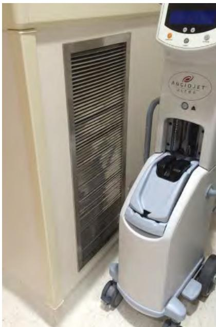
**Figure 6:** A louvered low-return grille in a cardiac catheterization laboratory room at Wheaton Franciscan Healthcare—Franklin in Franklin, Wis.
