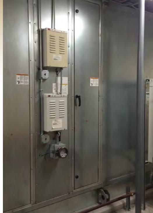
**Figure 5:** An electronic air filter is shown in a typical air handling unit at Wheaton Franciscan Healthcare—Franklin in Franklin, Wis.
