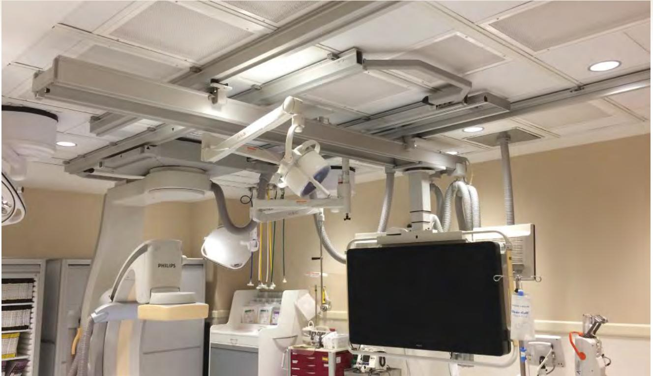
**Figure 2:** Laminar-flow supply-air diffusers are shown in a cardiac catheterization laboratory room at Wheaton Franciscan Healthcare—Franklin in Franklin, Wis.
