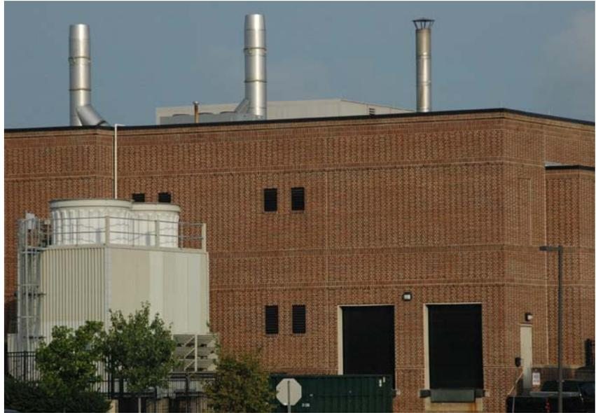
UVC-treated water produced by the air handlers during cooling season at the Delaware Biotechnology Institute on the campus of the University of Delaware is clean enough to be pumped into the cooling tower.
