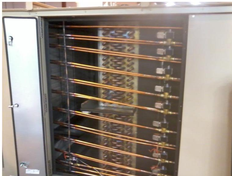
**Figure 1 – Controllable Wrap-Around Heat Pipe with Solenoid Valves (Model DHP-C)**
